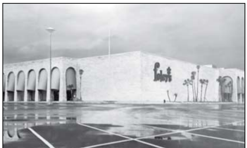
The above photo shows the Foley's Alameda Genoa store upon completion of construction. Longtime residents may remember the store's decorative turquoise awnings.
