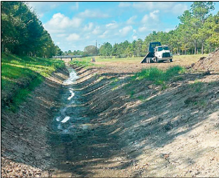
A FAST Team from the Harris County Flood Control District recently completed desilting a channel near the hike-and-bike trail on Blackhawk. Improved conveyance along the channel will help prevent local flooding.
