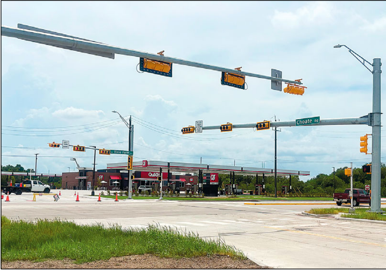
A new traffic signal was recently erected and activated on FM-1959/Dixie Farm Road at Choate Road near the Gulf Freeway. The signal is presumably to accommodate the incoming Quick Trip truckstop, which appears to be opening soon following months of
