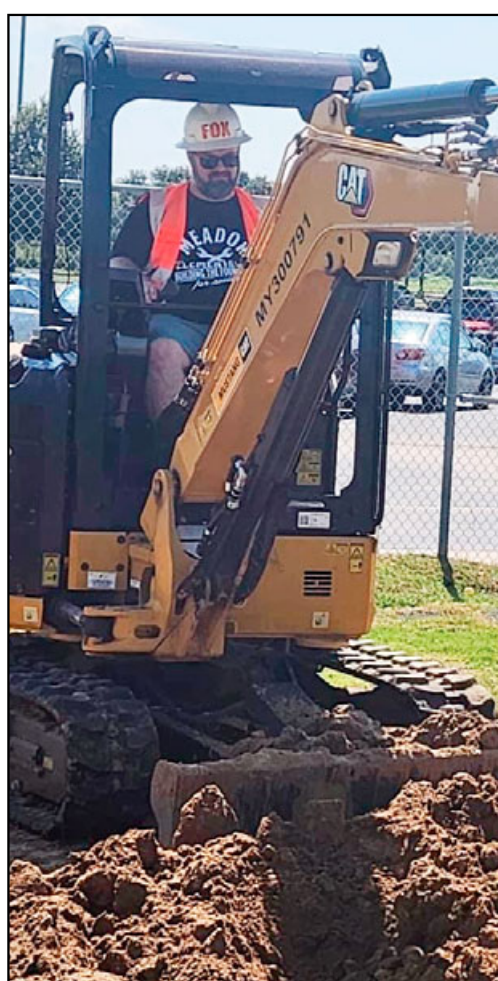
Kevin Fox, assistant principal, maneuvered a Cat mini-excavator.
