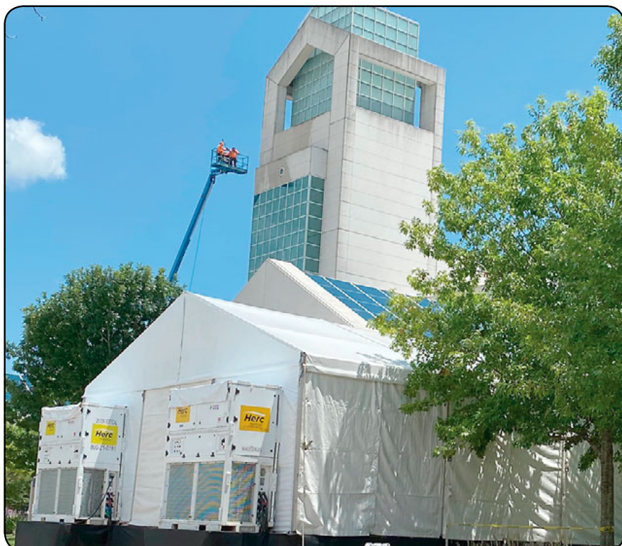
Memorial Hermann Southeast recently installed tents to handle overflow patients at the area facility. The measure takes place as the number of COVID cases continues to climb in the South Belt community. This past week, there were 500 new cases reported in just the immediate South Belt area. This marked the second time since the pandemic began that the South Belt community has surpassed the 500 mark in one week. Photo by Marie Flickinger
