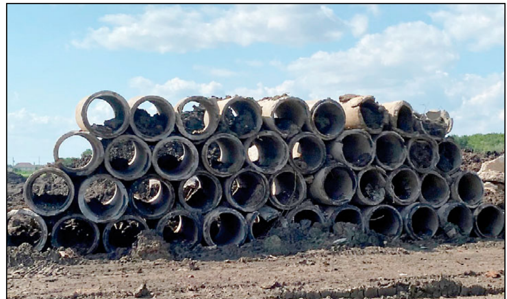
These drainage pipes, which previously drained Southbend subdivision are waiting to be taken out of the subdivision. The drainage project will greatly improve
