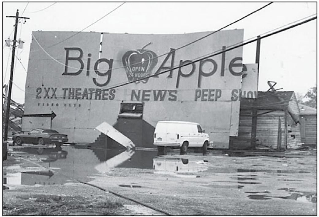
The Big Apple adult theater is shown above in 1983 after being struck by a tornado during Hurricane Alicia. Two years later, the controversial business was destroyed by an unsolved fire. See related photos on Page 1 and Page 4.
