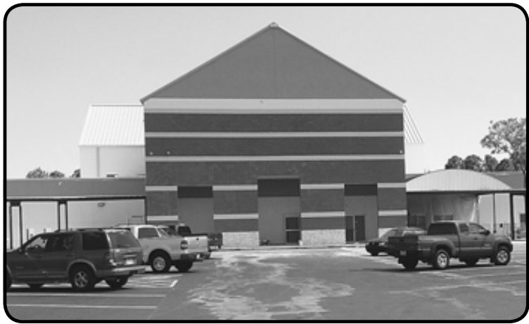
A massive new church is being constructed on Kleckley across from Almeda Mall in the pair of buildings that once housed the Marshalls and Target shopping centers. Originally founded in Nigeria, the Mountain of Fire and Miracles Ministries now reportedly has branches on every continent. The new location will serve as the organization's U.S. headquarters. Photo by James Bolen
