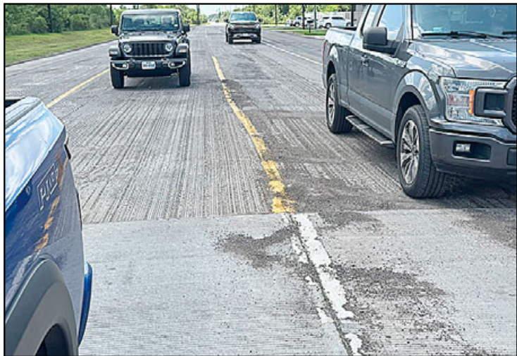
A city road improvement project is currently underway on Beamer between Dixie Farm Road and El Dorado Boulevard. See related story and photo on Page 1.
