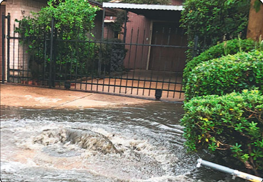
The residence above, located on Sagepark at Kirkfair in the Kirkwood South subdivision, has routinely had raw sewage spill from a nearby manhole into its yard and interior following heavy rains. Fixing the problem has proven difficult for the homeowner, as the problem is connected to infrastructure from the City of Houston and the Sagemeadow MUD. It is hoped that funds recently earmarked by the city for sewer system improvements will help rectify the problem. See related story this page. Photo by Marie Flickinger
