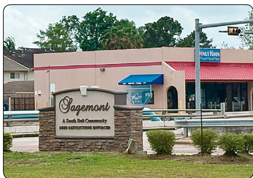
The Sagemont Civic Club recently repaired the subdivision's two-sided sign located near the intersection of Hughes Road and Beamer. The sign suffered extensive damage late last year when it was struck by an uninsured driver. The repairs were made possible through maintenance fund dues paid by Sagemont homeowners. The group hopes to make similar repairs on its other two smaller signs located on Hughes at Sageglen and on Hughes at Sagecanyon, marking the east and west entrances to the subdivision, respectively. Photo by James Bolen
