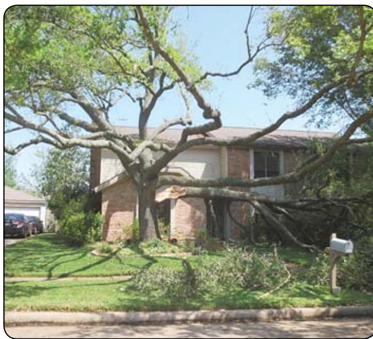
Winds caused a large tree limb to snap at a residence in the Sageglen subdivision, narrowly avoiding the home. Despite reports to the contrary, the damage was likely not caused by a tornado. Photo by Ann Abernathy
