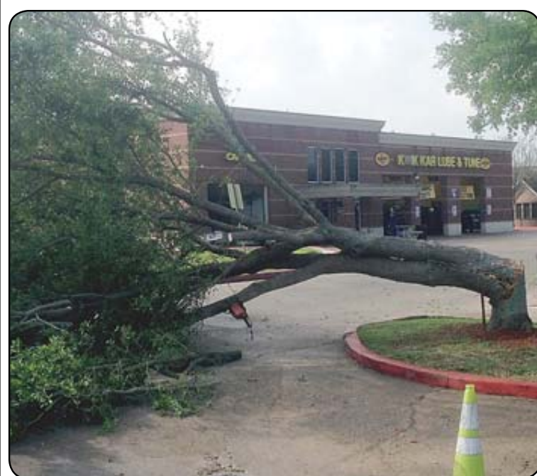
Strong winds snapped a tree in half at the Kwik Kar Lube Center & Ocean Wash in the 11200 block of Scarsdale. Multiple other nearby businesses also suffered extensive damage. Photo by James Bolen
