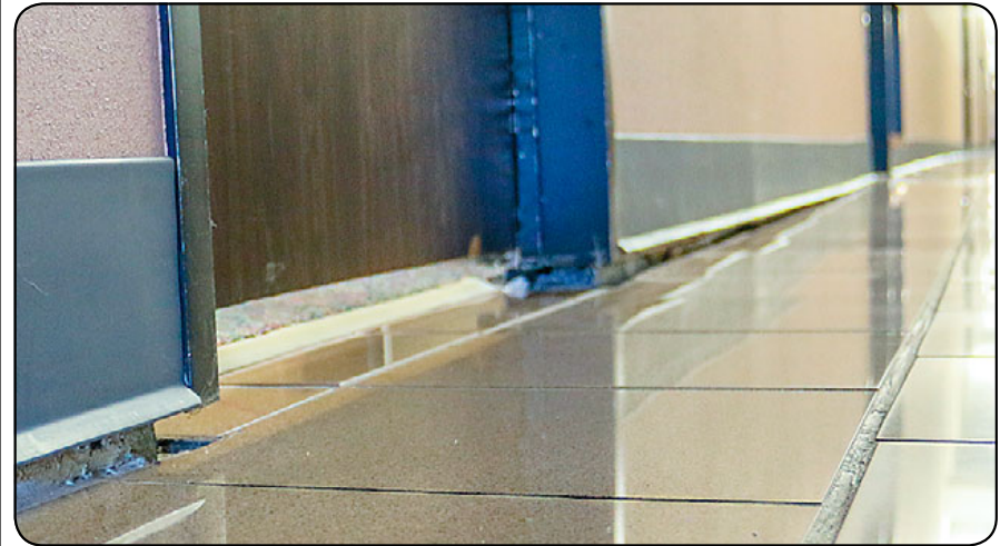
At its November meeting, the Pasadena ISD board of trustees approved the design and development phase of a new administration building to be located on Mickey Gilley Boulevard near Fairmont Parkway. Pasadena ISD officials say the facility is necessary because the existing building is aged, and making the needed improvements would not be cost effective. Above, the wall is shown separating from the flooring at the existing administration building.
