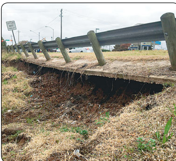
A collapsing guardrail on the southbound lanes of Beamer just north of Scarsdale has concerned many South Belt residents. The collapse seems to be caused by ground eroding near the road. Harris County officials have deemed the problem an emergency and said it would be addressed in the next one to two weeks. See related photo on Page 1A.
