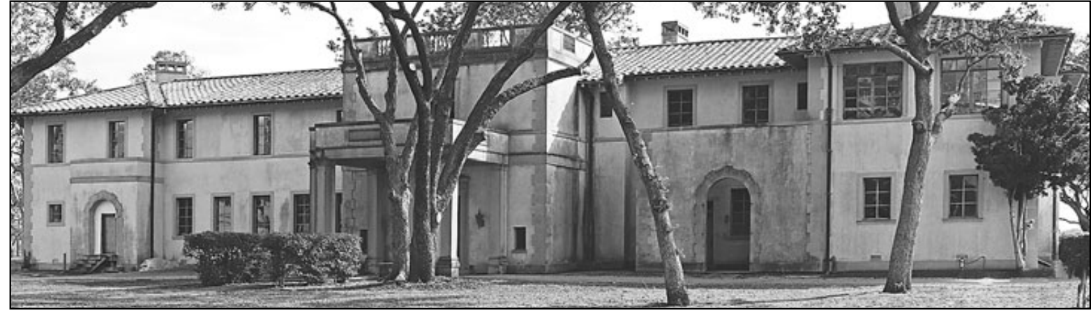
Above is the West Mansion as most have seen it; upper right photo shows the landmark that was recently demolished.
