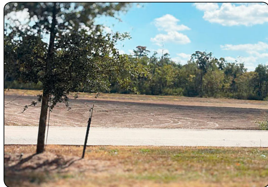
Work continues on the Friendswood Regional Stormwater Detention Basin, with preliminary excavation recently coming to an end. To be located near FM 1959/Dixie Farm Road and Blackhawk Boulevard (see map on Page 2), the basin is expected to assist in local flood control by detaining approximately 700 to 1,300 acre-feet in stormwater storage, once complete. The project is now currently in the design phase, with an expected completion date in late 2026.
