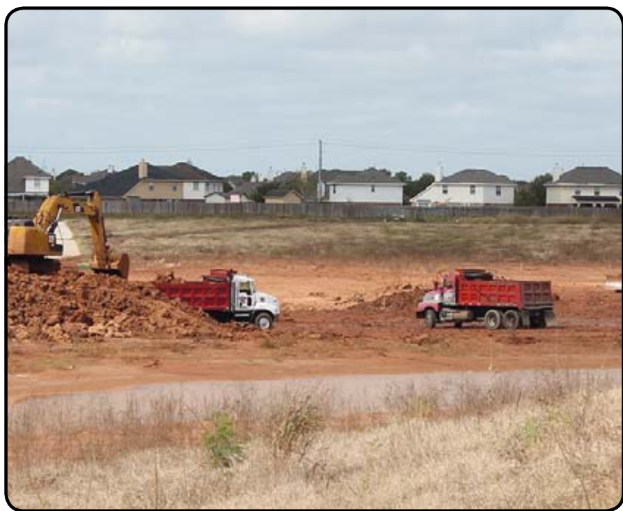
Work on the South Belt Stormwater Detention Basin is moving forward, with crews now working on Phase II of the project. Located in the former Southbend subdivision, the pond will hold roughly 400 million gallons of stormwater once completed. Crews are shown above hauling dirt from the site to an approved county dump. Photo by Marie Flickinger
