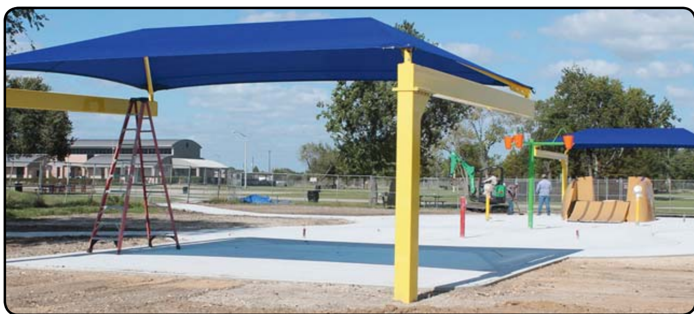
Work recently began on a splashpark at El Franco Lee Park. The 2,700-square-foot structure will include a splash deck, a mushroom maze and flower sprinklers. The splashpark was the last project the late El Franco Lee promised the South Belt community before his death this past January. Construction of the splashpark is expected to complete next month. Photo by Marie Flickinger
