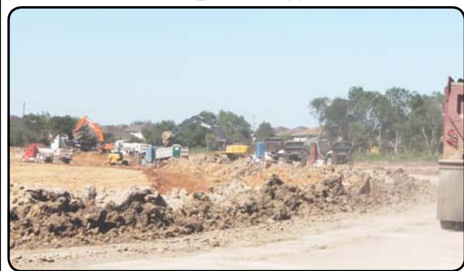
The Leader has received multiple calls regarding construction taking place north of Hall Road behind the H-E-B located at Blackhawk and Beltway 8. The work involves constructing a holding pond associated with the ongoing project to widen Beltway 8. The retention pond is one of many planned that are related to the endeavor. Photo by Marie Flickinger
