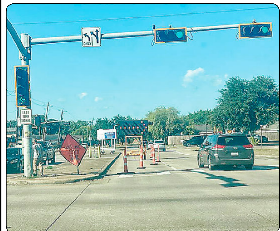
A Houston District D project is currently underway to make roadway improvements to Beamer north of Beltway 8. According to District D officials, scheduled work involves making mill and overlay improvements along the area thoroughfare from Beltway 8 to Fuqua. The endeavor is similar to another District D project that recently made such improvements on Beamer to the south between Dixie Farm Road to El Dorado Boulevard.
