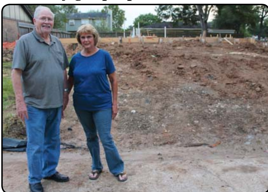
William and Kathleen Tullis (shown above) are among a group of four homeowners trying to block the proposed construction of a duplex in the Woodmeadow Section I subdivision, located at 11502 Quincewood Drive at Olivewood. The homeowners contend the structure violates the neighborhood's deed restrictions. The subdivision, however, lacks a homeowners' association to enforce the restrictions, prompting the group to hire its own attorney.
