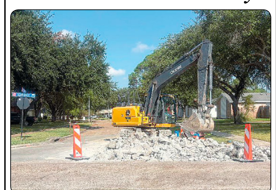
A county crew is shown above making street repairs on Scarsdale near Sagewind in the Sageglen subdivision. The project is just one of multiple road repair endeavors currently underway simultaneously in the area. The street improvements are part of a plan launched by Precinct 2 Commissioner Adrian Garcia to make repairs to damaged panels along thoroughfares on roadways in unincorporated parts of the South Belt community.
