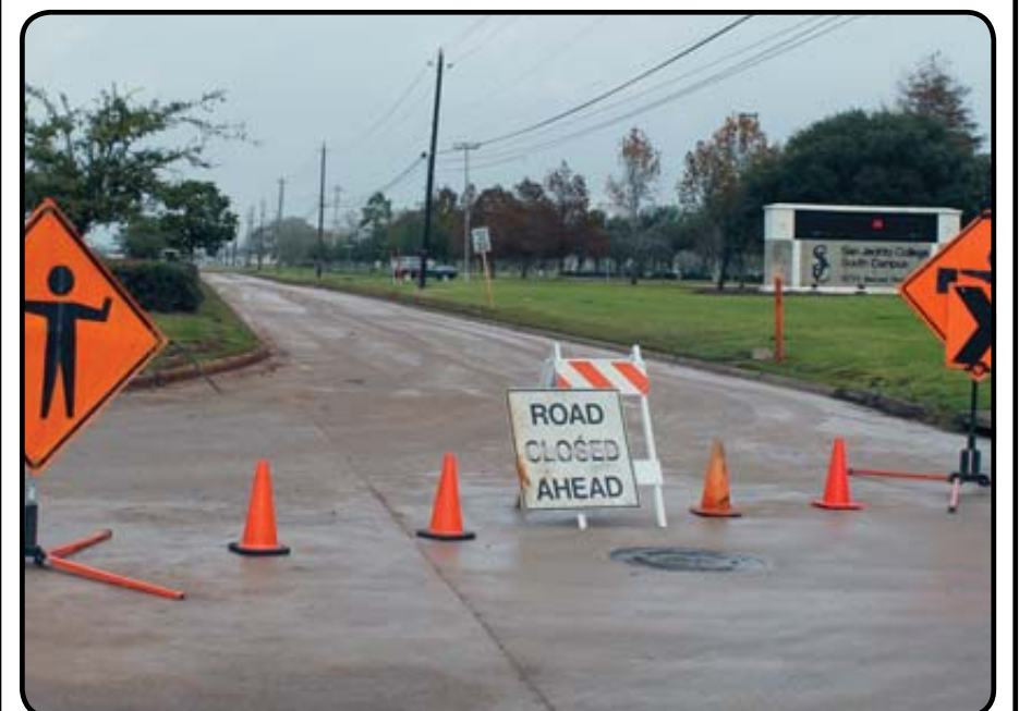
South Belt residents have undoubtedly noticed the constant stream of dump trucks driving up and down Beamer, Beltway 8 and Blackhawk in recent weeks. This trend is expected to continue through 2017 and much of 2018. The trucks are hauling dirt from the site of the future detention pond near Beamer and Dixie Farm Road to a dump site near Beltway 8 and Mykawa. Mud from the trucks recently caused the closure of Beamer, forcing traffic to divert through San Jacinto College South (shown above). Photo by Marie Flickinger
