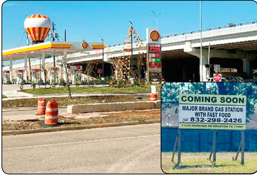
After months of construction, the new Shell service station located on Beltway 8 at Hughes Road/Sabo opened to the public. This marks the third gas station to be located at the area intersection, with signage for a possible nearby fourth station to be located on Hughes Road at Sageglen where the Church's Chicken was once located (see inset photo). Photos by James Bolen
