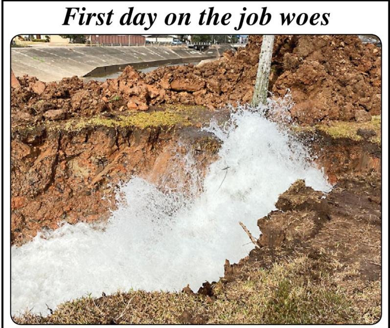
Work crews from Complete Concrete working for the Harris County Flood Control District Tuesday broke a city water main, as they began construction on drainage improvements along Beamer Ditch. The incident took place between Highland Meadow Drive and Sagedowne. The \$10.7 million project will make improvements from Sagerock to near Dixie Farm Road. Work on the project is expected to take two years to complete. Photo by Marie Flickinger
