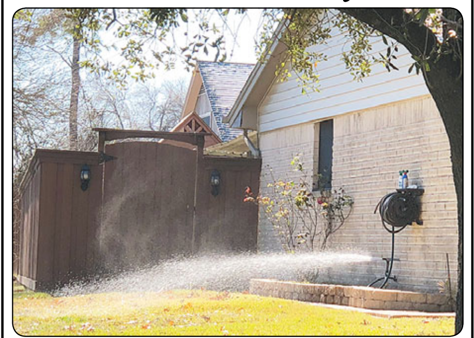
A malfunctioning water spigot outside a home on Kirkshire at Beamer was spraying water onto the area thoroughfare, causing dangerous driving conditions Wednesday, Jan. 17. While Wednesday was free from precipitation, temperatures were still below freezing, creating a hazard. Several residents attempted to make contact with the homeowner to no avail, as no one answered the door, despite there being two cars in the driveway.
