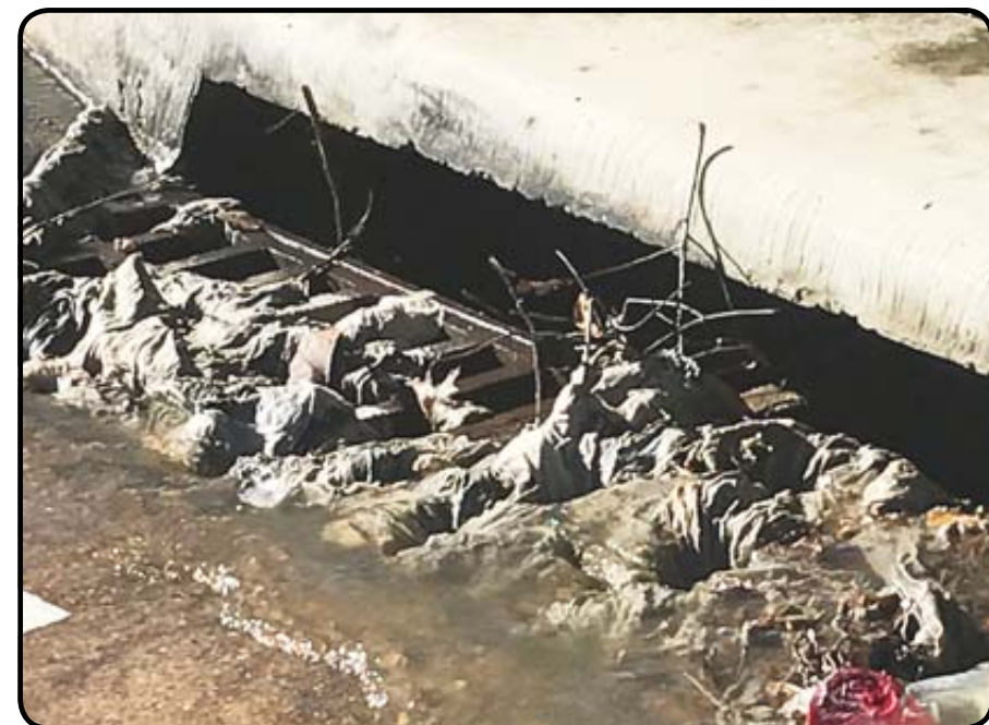
Multiple Sagemont residents, primarily on Sagedowne near Sageglen, recently complained of raw sewage overflowing in and around their homes following heavy rains. Sagemont Civic Club President Kay Barbour said the issue dates back more than 20 years. She is currently working with city officials to fix the problem. Shown above is a storm drain at the aforementioned intersection clogged with sewage debris. Photo submitted
