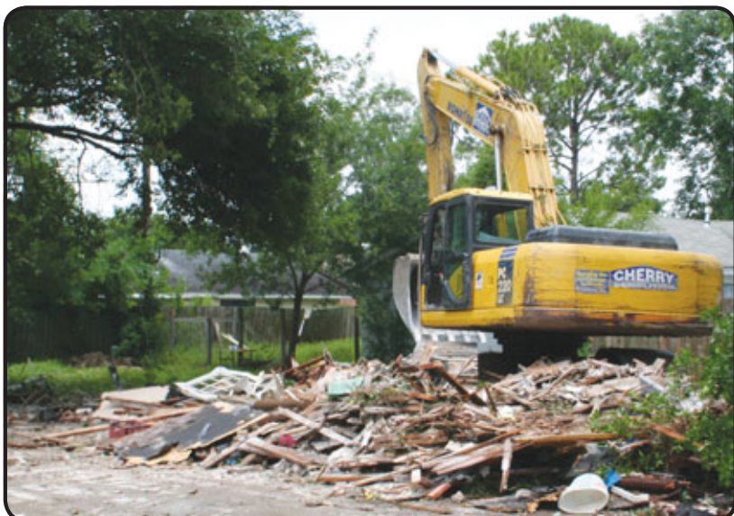
Two homes in the 11500 block of Sagedowne were demolished Thursday, June 4, as the result of a government buyout due to repeated flooding. Several other homes on the street have been leveled over the last decade. Many Kirkwyn residents in the Kirkwood subdivision would like to have their homes bought out if necessary repair work is not done to alleviate their flooding problem. Photo by James Bolen
