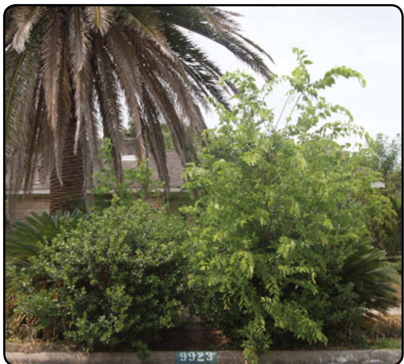
The above house and its unkempt lawn located at 9923 Sageroyal has drawn the ire of several Sagemeadow residents. According to neighbors, the house has been abandoned for at least two years. Although uninhabited, the house, owned by Jeffrey and Arlene Rittmer of Baytown, is current on all of its taxes. The matter has been turned over to Harris County officials.
