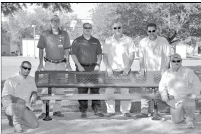
San Jacinto College South facilities and construction team members installed new benches and landscaping for one of the campus' main areas. Pictured are, left to right, Rene Amaro, Terry Ballard, Ron Andell, Jeff Tschappatt, Troy Freeman and Jose Montoyo. Photo by Andrea Vasquez
