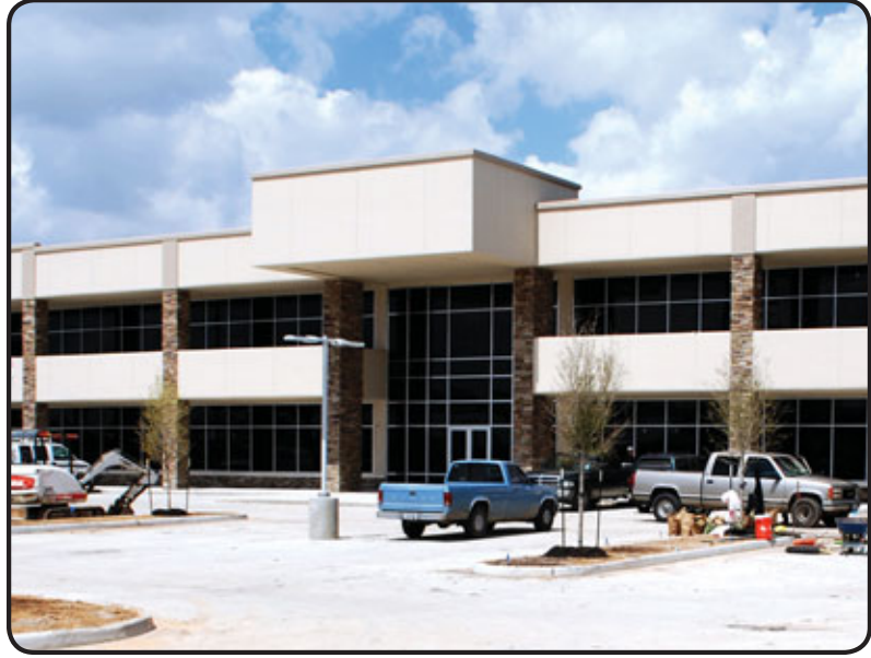
As of press time, FCT Capital Partners LLC and local State Farm insurance agent Norwood Richardson were the only tentative occupants of the nearly completed office building on the Gulf Freeway near Fuqua. Construction crews were seen on site, but external work on the building's front had been finished. Photo by Matt Griesmyer
