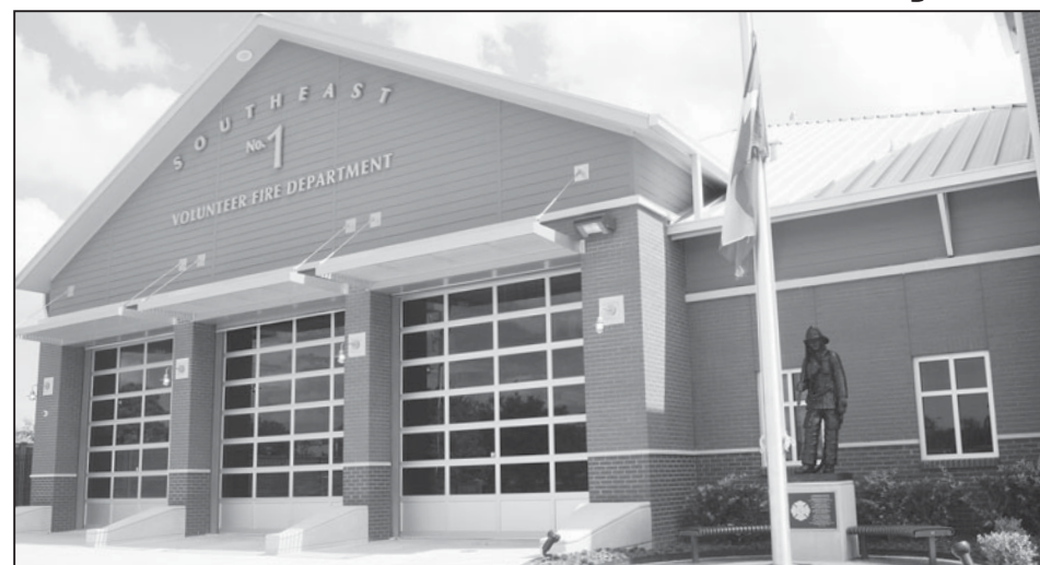
New Southeast Volunteer Fire Department station #1 located on Scarsdale Boulevard
