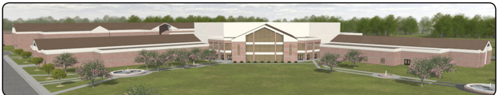
Sagemont Church recently broke ground on its new sanctuary and adult education center. Part of the church's "living proof" project, the structure will occupy 120,000 square feet and hold 2,500 people. The construction will take anywhere from 18 to 24 months to complete,
