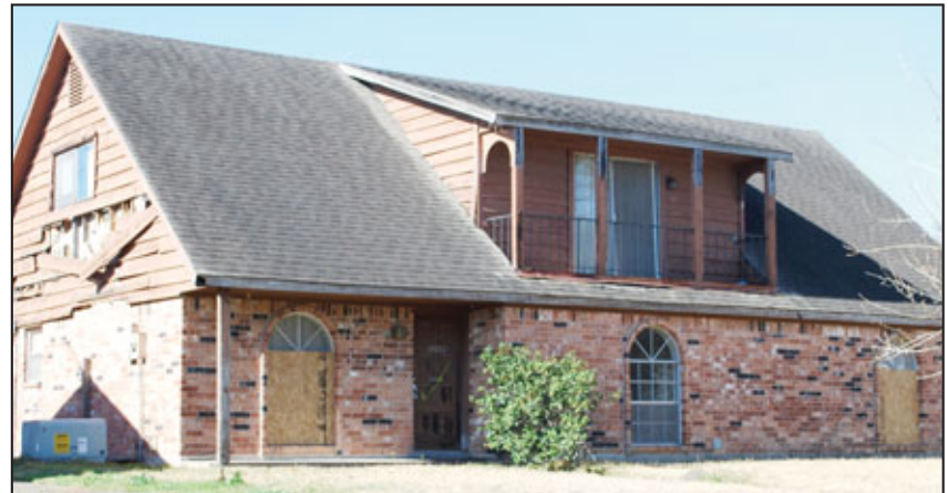
This vacant house at 11002 Sageburrow was boarded up by city officials.
